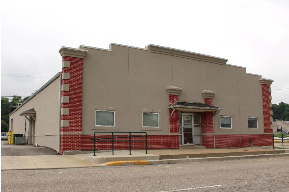
Bulldog Battery – 98 E. Canal Street - COMPLETE
