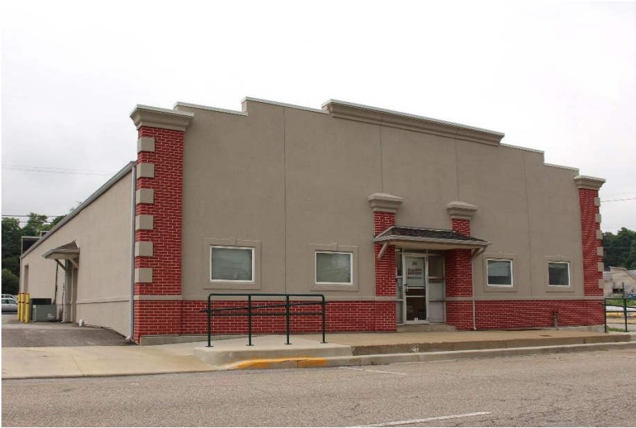
Bulldog Battery – 98 E. Canal Street - COMPLETE
